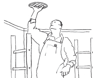
Fitting extractor louvre in ceiling
